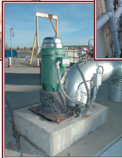
Primary Clarifier Scum
