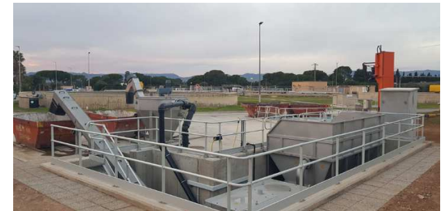
Sewer Grit Receiving Station
